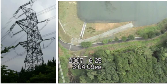
Fig.6 High Voltage Electrical Power Facilities
