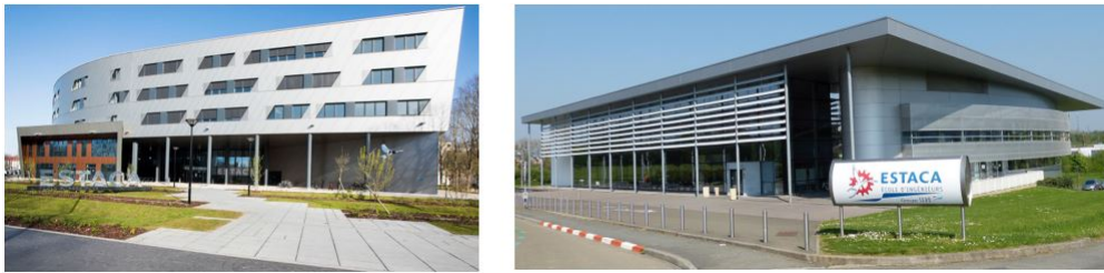
Figure 1: ESTACA in Saint-Quentin-en-Yvelines (left) and in Laval (right)
